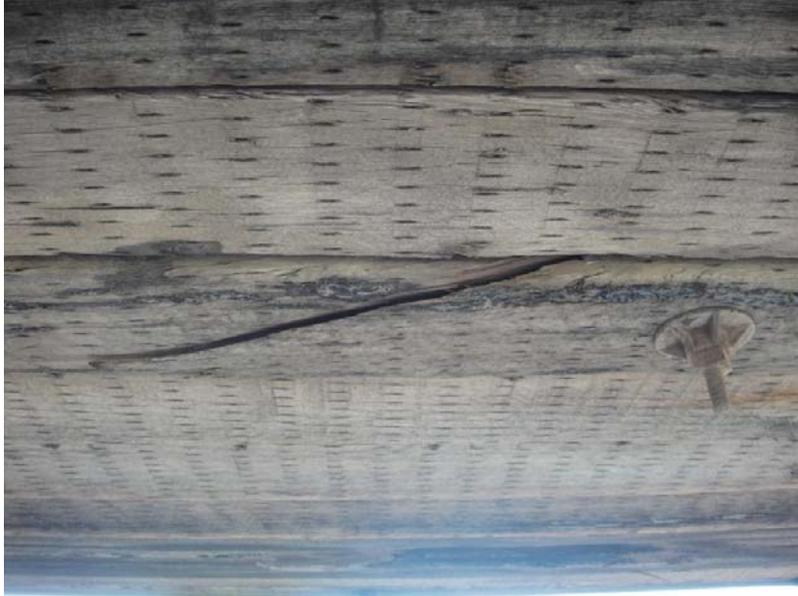
**Figure 6 – BRG 875.7 – Broken Stringer To Be Replaced**
