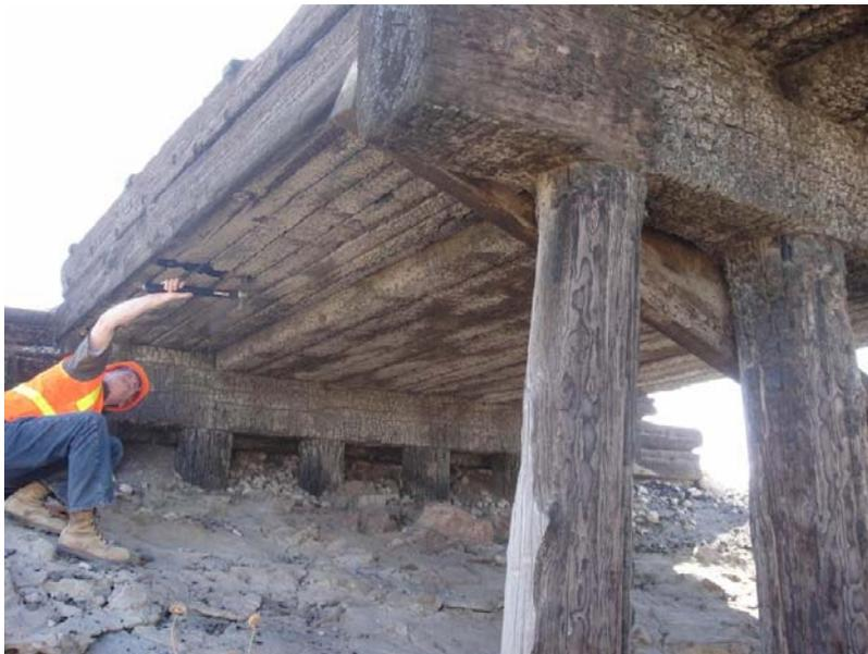
**Figure 7 – BRG 877.6 – Fire Damaged Bridge To Be Replaced**
